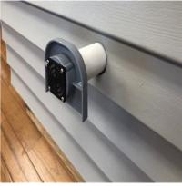
A thicker walled structure like tiny houses have insulation, wood walls, and siding that would require a space extender through the wall to attach the vent and the hose. We use a 1-1/4" PVC to make this extension.
